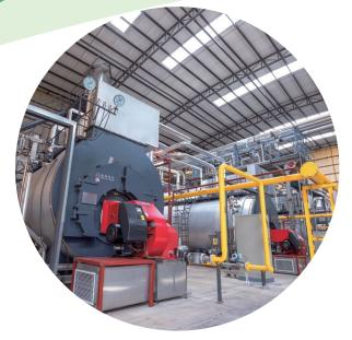
▲ 天然氣鍋爐提供生產能源 Power supplied by natural gas boilers
