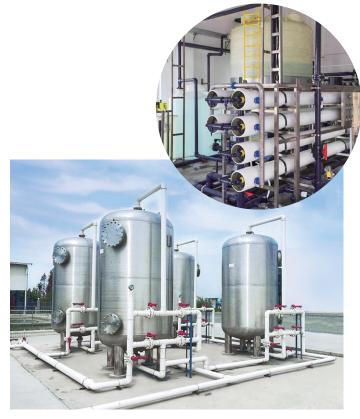
▲ **中水回用系統**處理污水可再用 Greywater Recycling system to recycle treated wastewater
